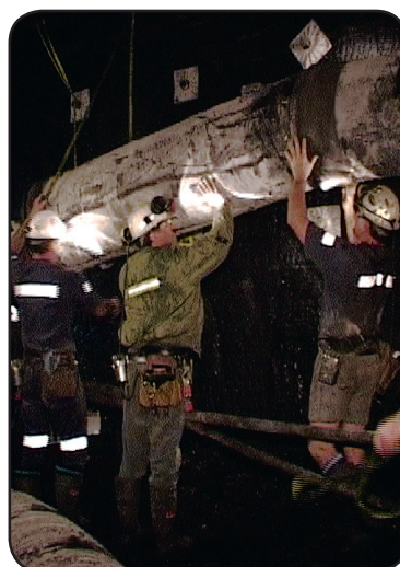
Installing vent tubes
